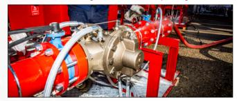
each one provided with its own diaphragm and actuation trim, which offer two independent waterways to the water spray system. Each priming chamber provides the nominal design waterway for the fire protection system: in case of failure of one diaphragm, the opening of the other diaphragm allows the hydraulic waterway for the correct operation of the water spray system.
