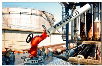
double channel hosting the rotational spheres. Shaped to keep the concentrated pressure losses to a minimum, the casting has a double internal waterway and can be used for water or water foam solutions. Addressing the specific requirements for harsh industrial environments & offshore applications.
