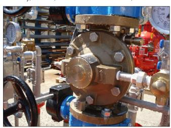
The materials of construction make SA Fire's series of deluge valves suitable for being used with sea water or water foam solution within harsh industrial environments & offshore applications. The cover plate on the VD and the cover plates on the VDD allow in-line maintenance and field replacement of the diaphragm.
