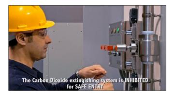
space. Lock off and shut off units are devices used to isolate the SA Fire HP Carbon Dioxide fire extinguishing system when personnel are required within the protected spaces. The lock off unit is installed upon the main entrance of the protected space while the shut off is installed on the pilot cylinder actuating circuit.
