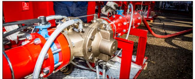
each one provided with its own diaphragm and actuation trim, which offer two independent waterways to the water spray system. Each priming chamber provides the nominal design waterway for the fire protection system: in case of failure of one diaphragm, the opening of the other diaphragm allows the hydraulic waterway for the correct operation of the water spray system.
