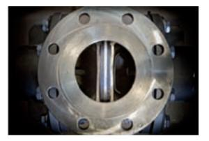
To carry out maintenance/repair on a VDD deluge valve, the operator begins by unlocking the isolation system of one of the two chambers.
