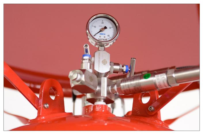
switches, monitoring system pressurisation, activation and discharge. Level Controls can be used for halocarbons to monitor gas leakage. The contacts are then hardwired in a local JB and use a cable turnbuckle to exit the tank zone. Outside the tank there is an Ex ia JB with I.S. barriers used to interface with dedicated F&G or with other
